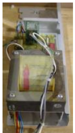
Power Supply and Transformer for HP 5890 GC
